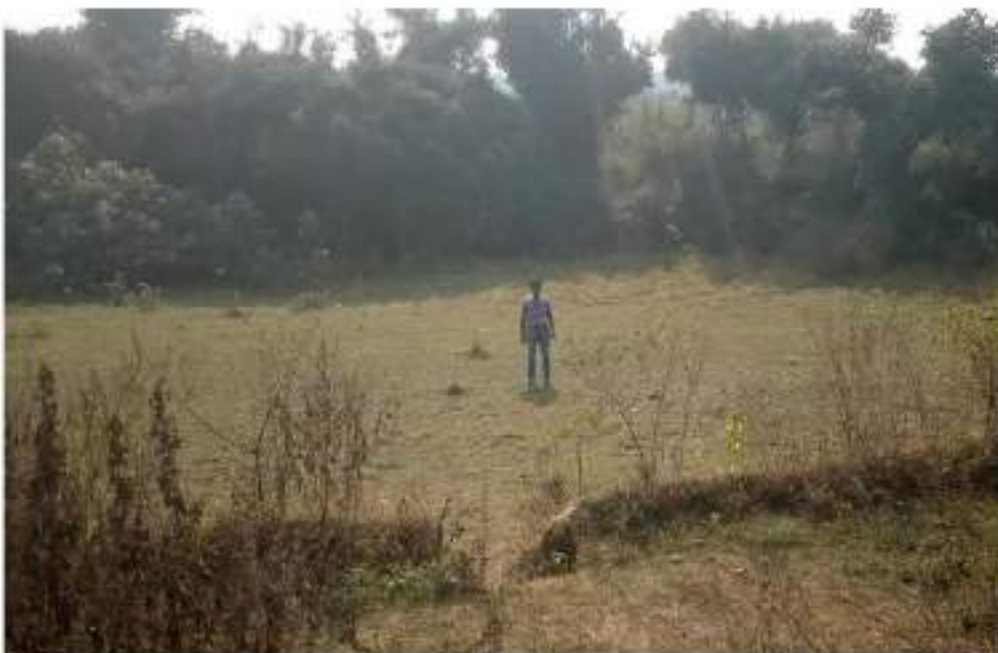
Figure 18: Sagged area due to subsidence, south of Block II OCP. (point 1 in figure 14 and table 5)
