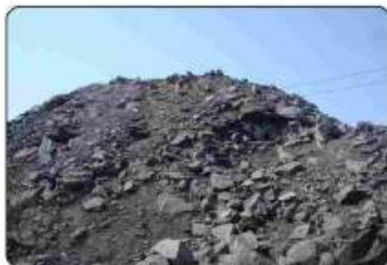
Over burden dump with 70° slope
