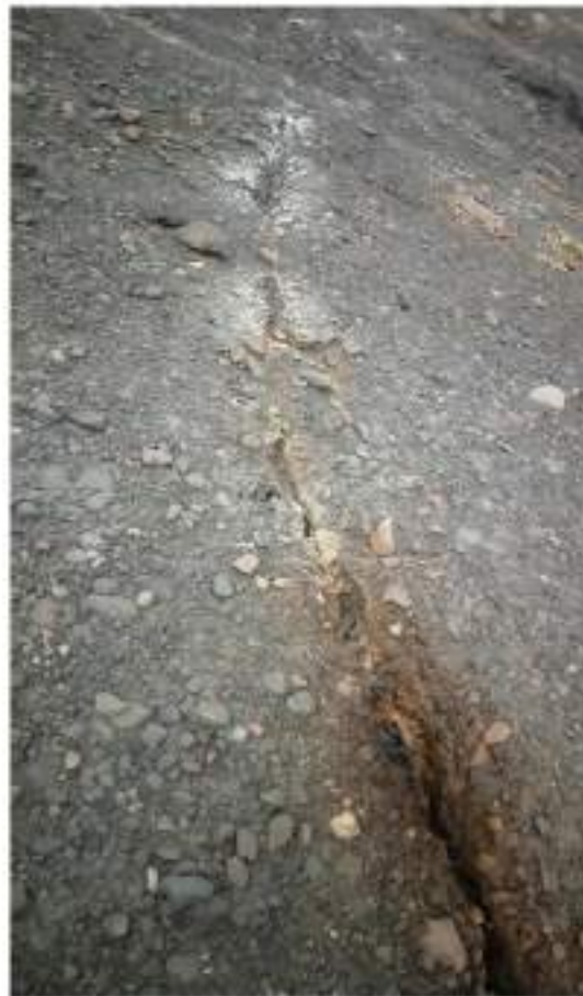
Figure 20: Fume cracks in the Bhulanbarari area.
