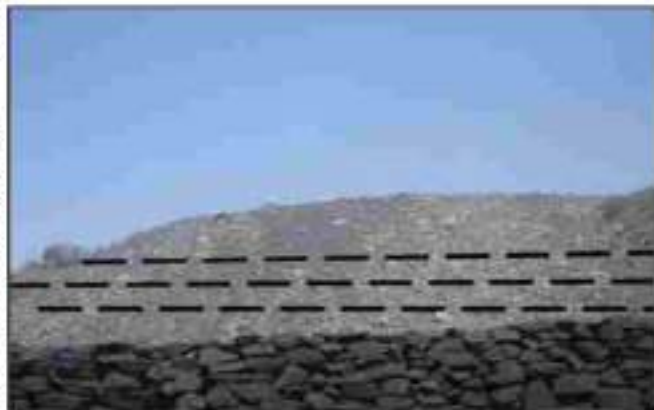
Plate 1b. Staggered contour trenches
