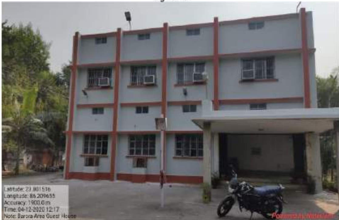
Proposed Rain Water Harvesting Site Barora Area Guest House, Cluster-I, Barora Area
