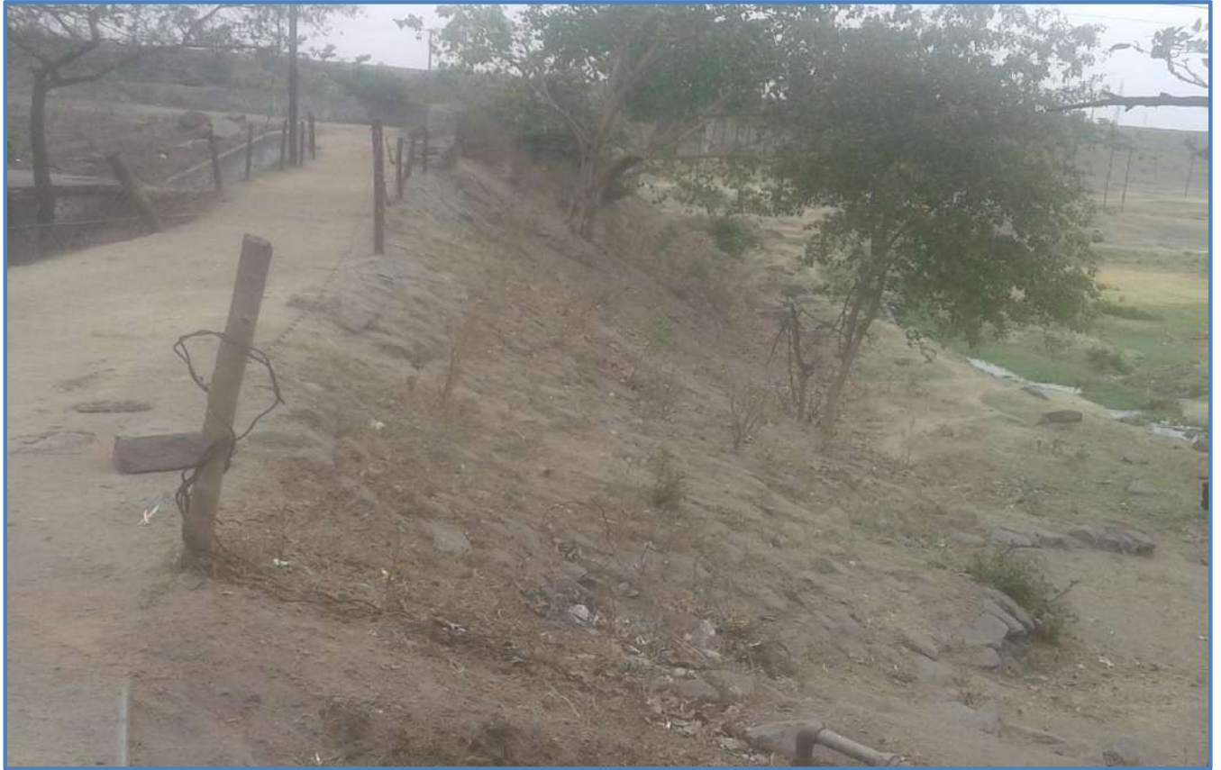
Picture 3 - Stone Pitching/embankment at Kari Jore
