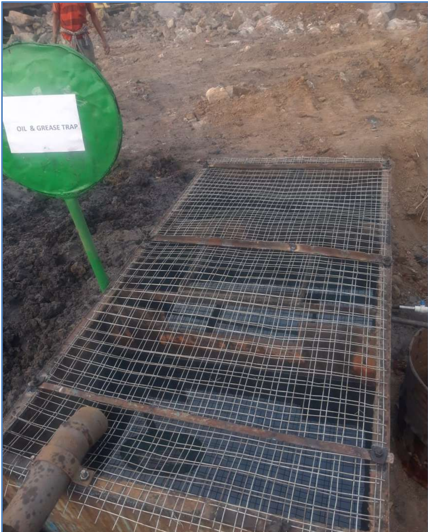
Picture 5 – Oil & Grease Trap
