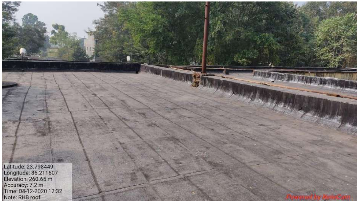
Proposed Rain Water Harvesting Site Regional Hospital Baghmara, Cluster-I, Barora Area
