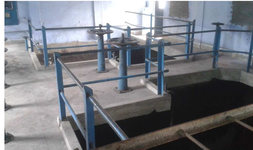
B. Units of Filter Plant
