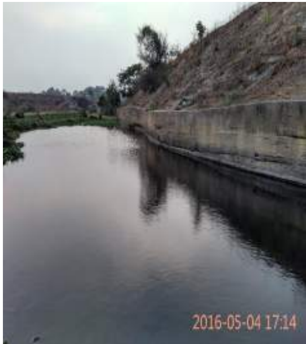
Pic 1- Toe wall with stone pitching at AARC
