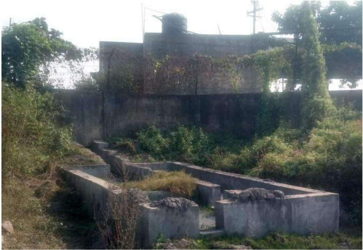
Oil & Grease trap at Nichitpur Workshop in Sijua Area.
