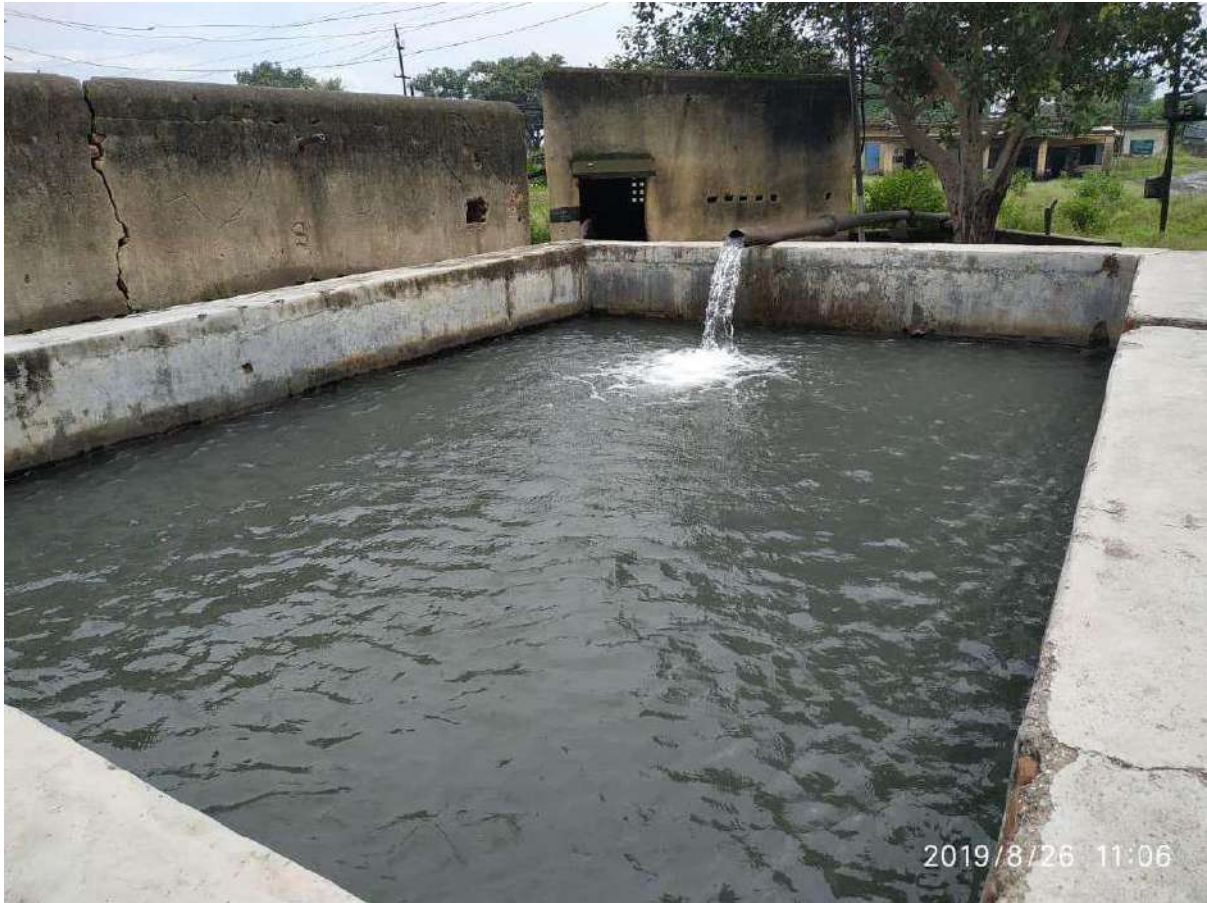
Sedimentation ponds and settling tanks for mine water utilization
