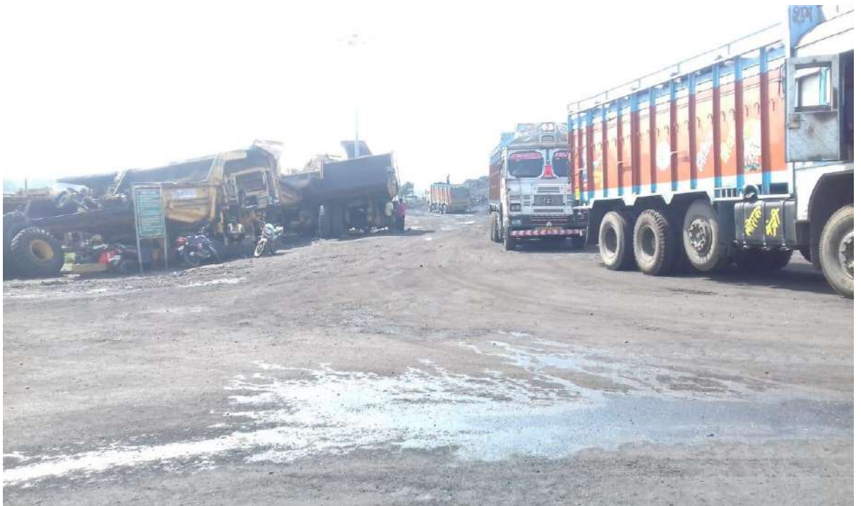
Roads constructed within colliery premises
