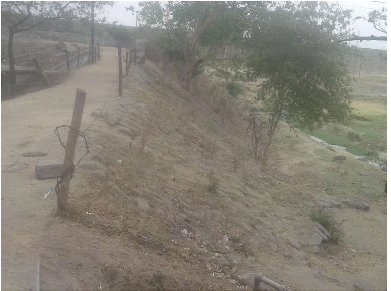
Figure 1 Stone Pitching/embankment at Kari Jore near Godhur Colliery.
