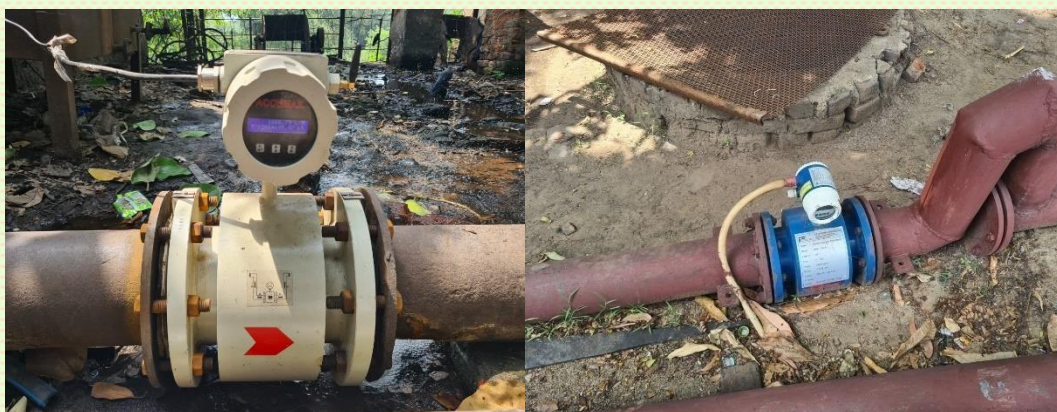
Digital Flow meters installed in BCCL
