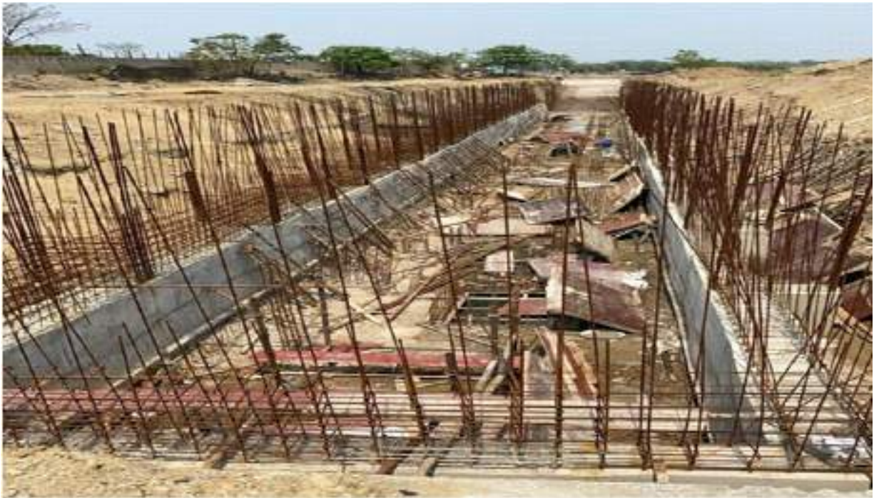
Construction of Raw Coal Receiving Track Hopper
