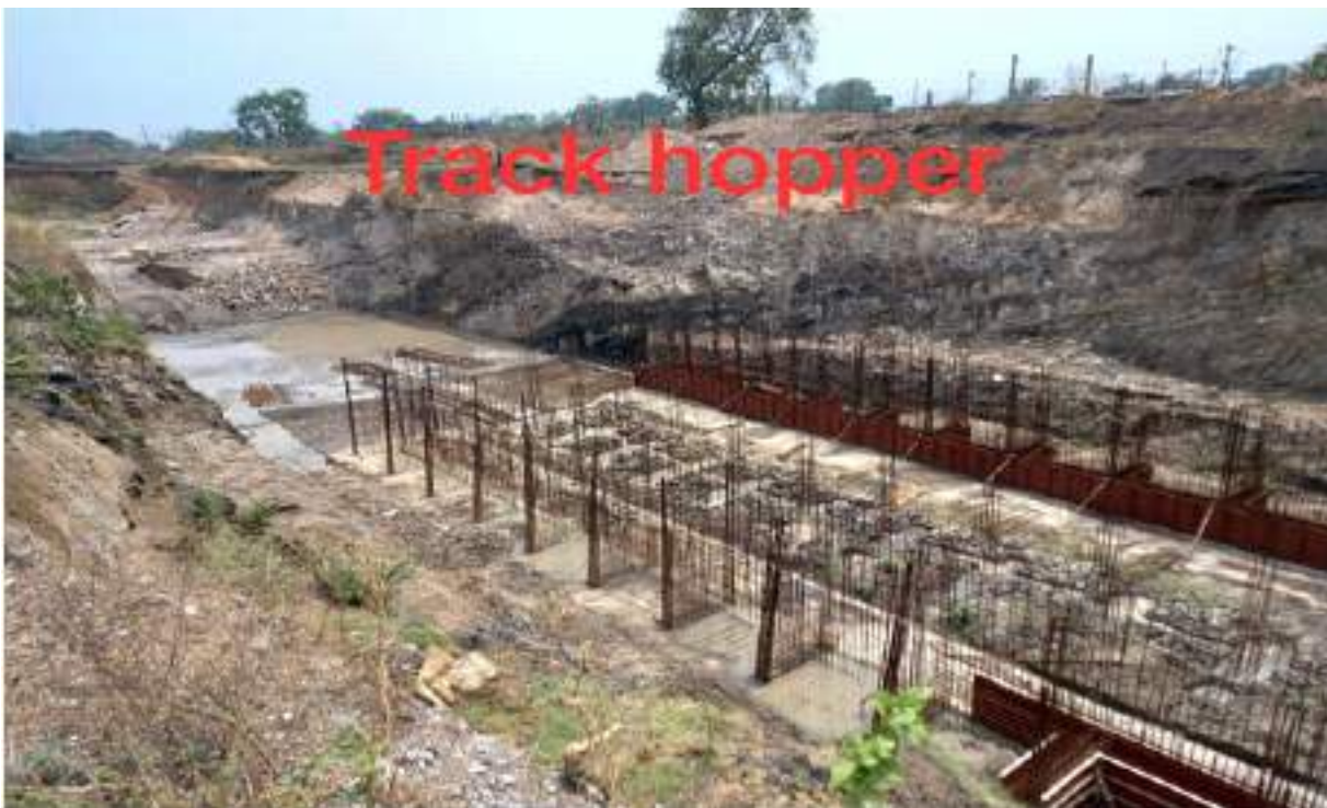
Construction of Raw Coal Receiving Track Hopper
