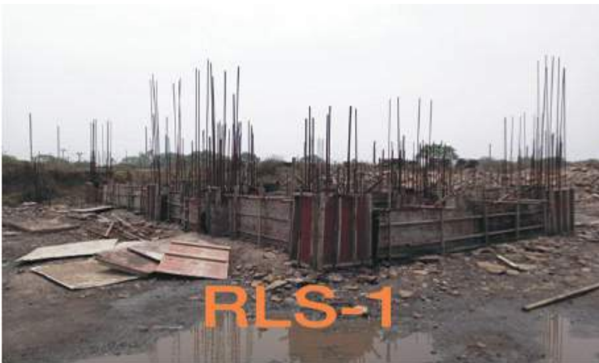
Construction of Rapid Loading System- 1
