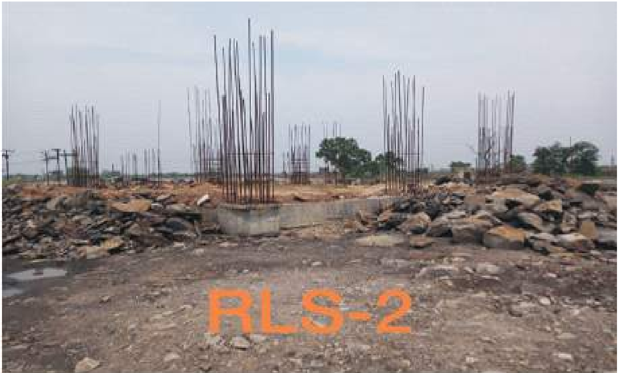
Construction of Rapid Loading System- 2
