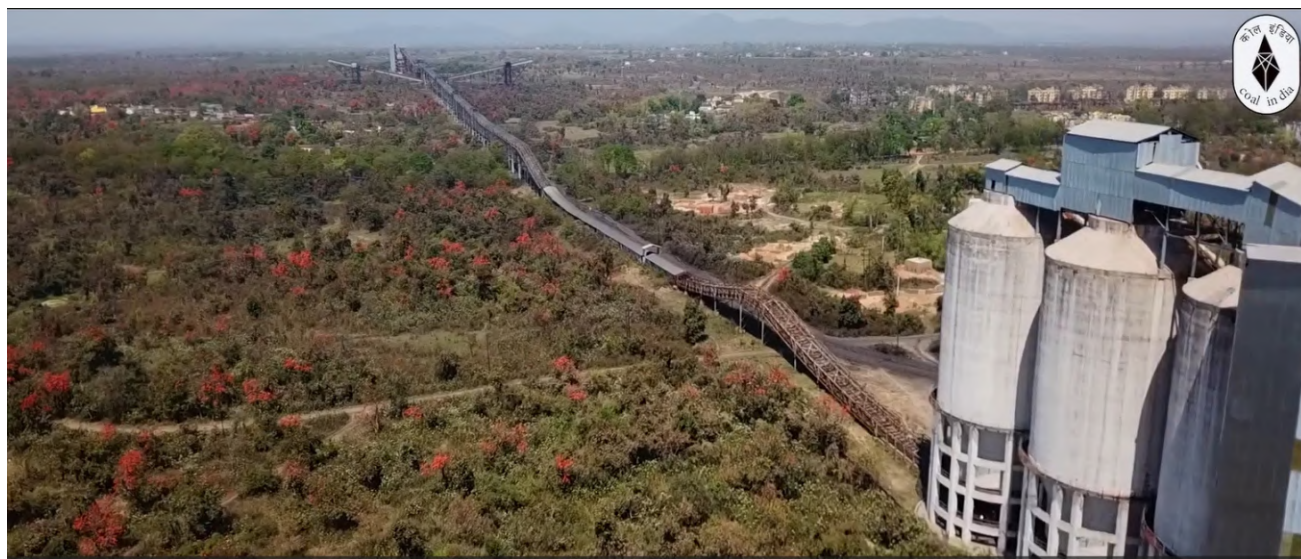
2.0 Mtpa Bhojudih washery under construction
