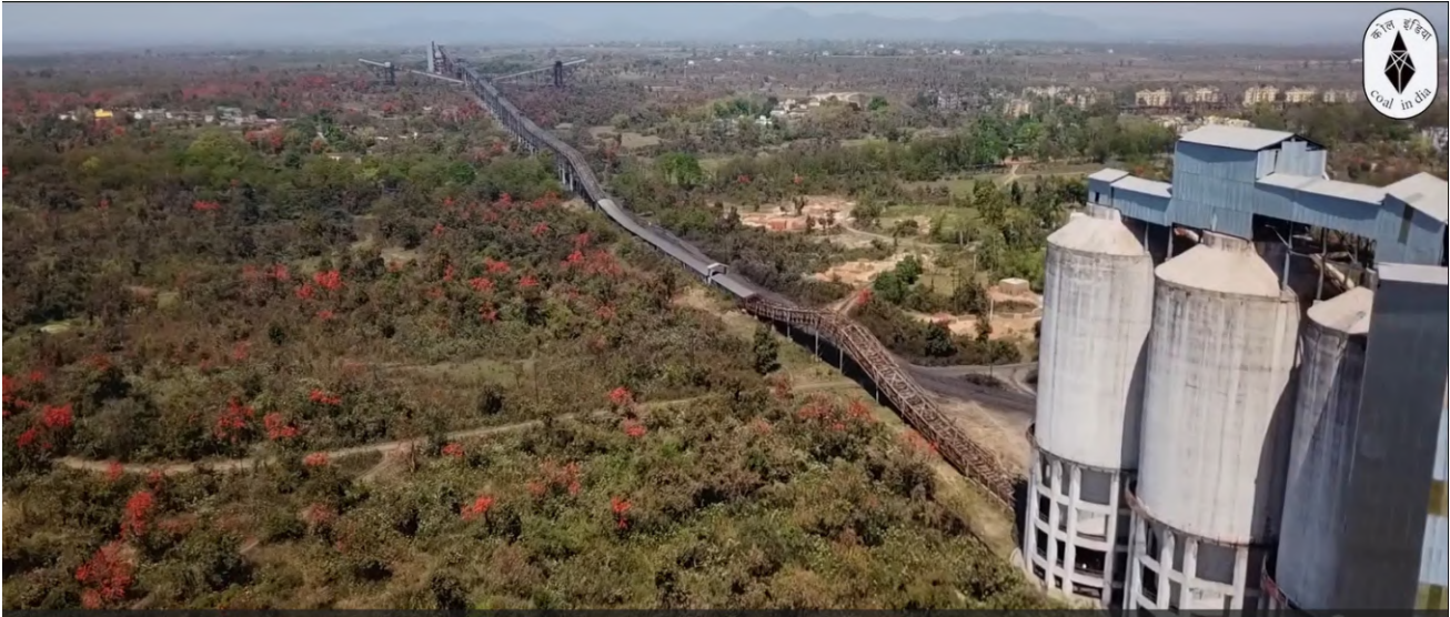
2.0 Mtpa Bhojudih washery under construction
